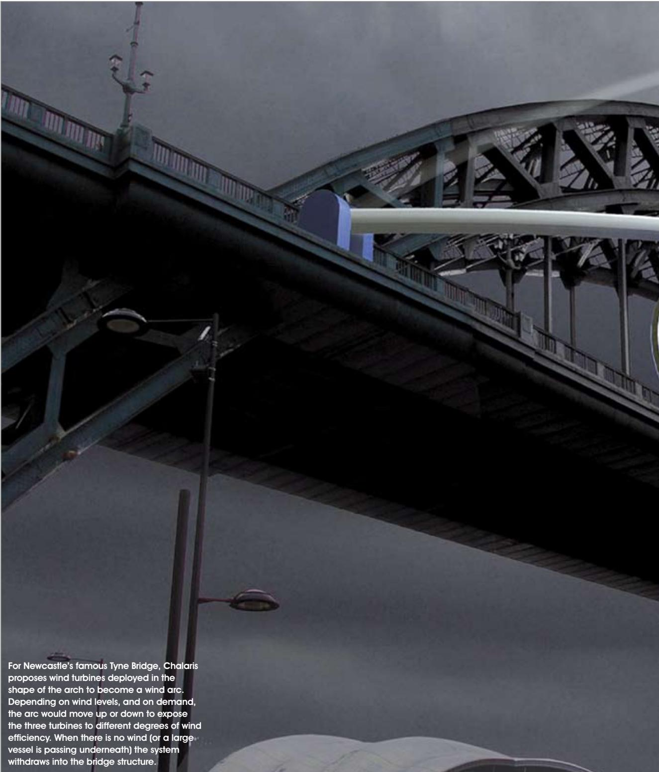
For Newcastle's famous Tyne Bridge, Chalaris proposes wind turbines deployed in the shape of the arch to become a wind arc. Depending on wind levels, and on demand, the arc would move up or down to expose the three turbines to different degrees of wind efficiency. When there is no wind (or a large vessel is passing underneath) the system withdraws into the bridge structure.
